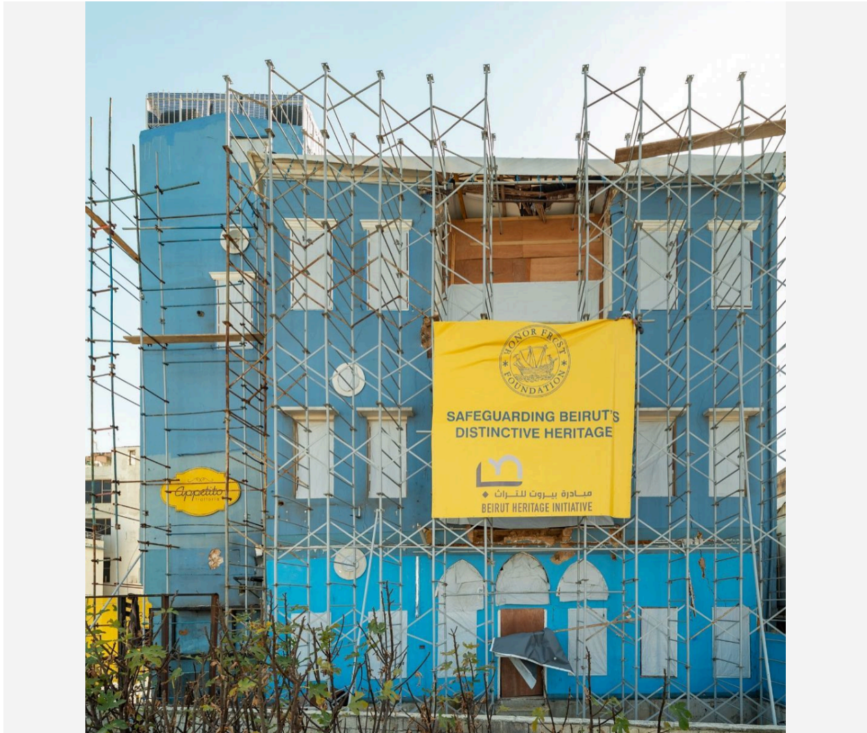
BHI's renovation of the Blue House
