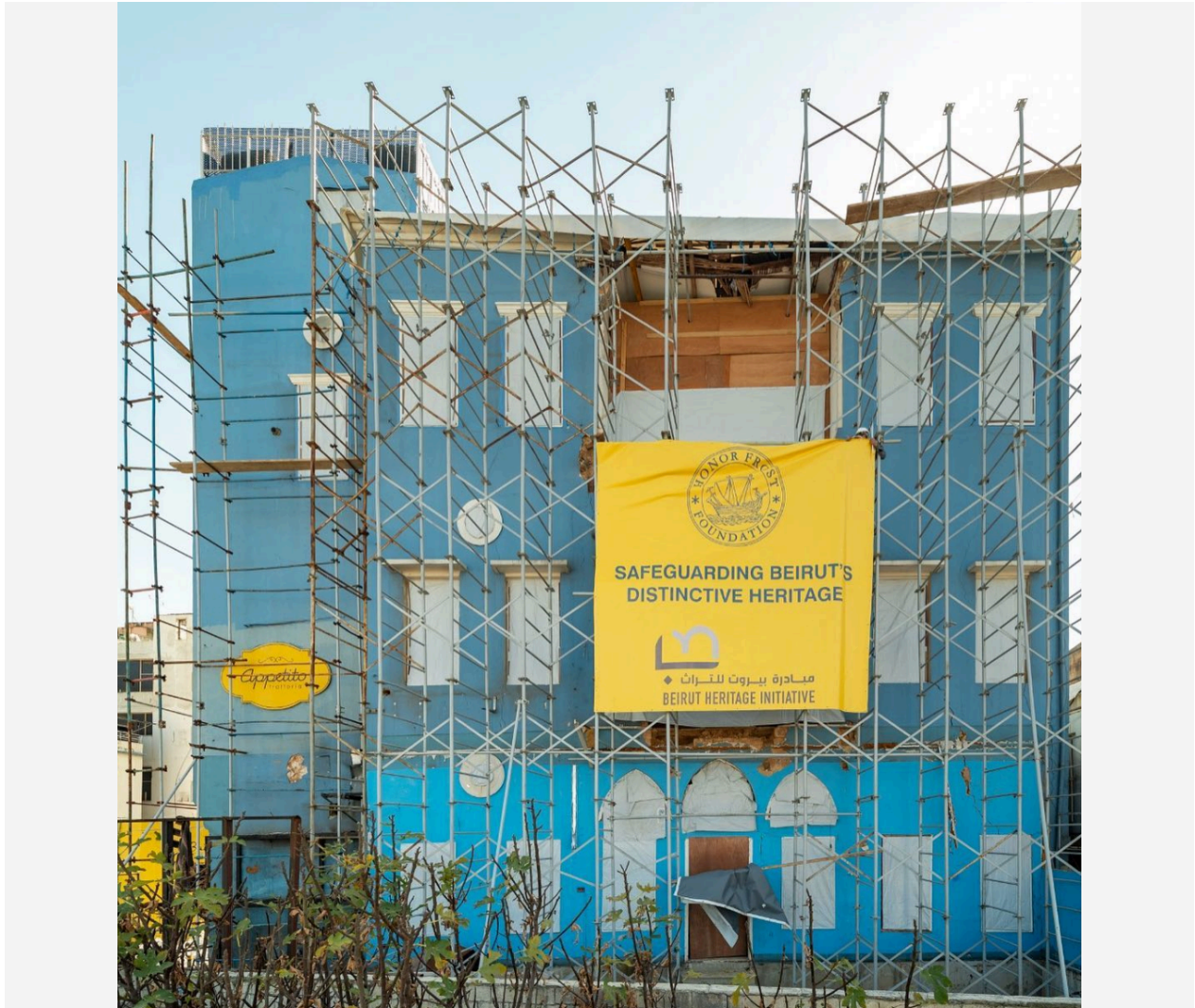
BHI's renovation of the Blue House
