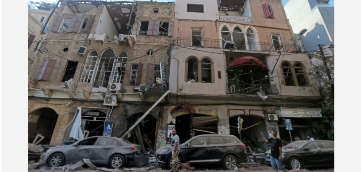
Pedestrians walk past damaged historic buildings on August 5, 2020, in Beirut's Gimmayzeh district which was heavily damaged by the powerful explosion that tore through Lebanon's capital [Getty Images]
