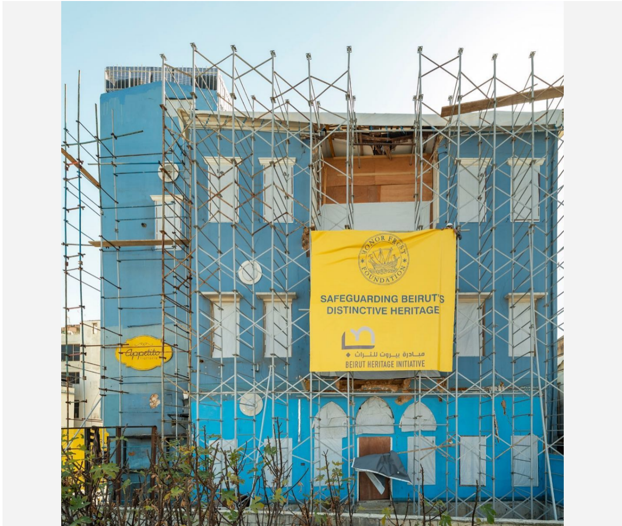
BHI's renovation of the Blue House
